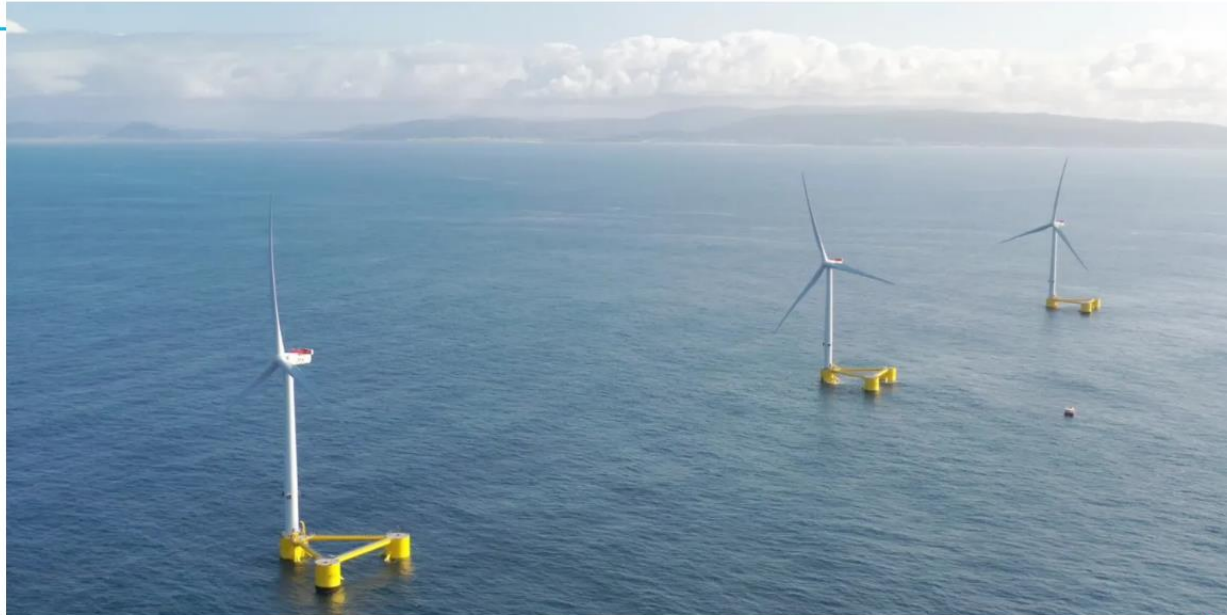
Photo: WindFloat Atlantic
